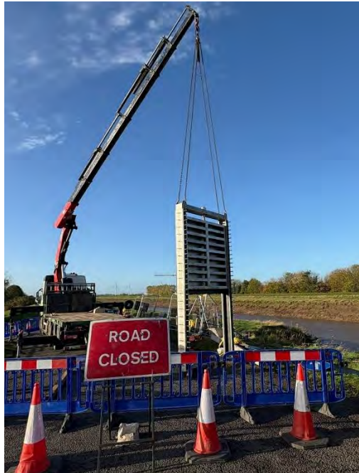
New penstock being lifted in
