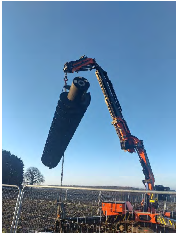
New screw pump being lifted in
