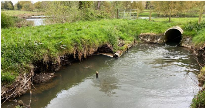
Culvert and bank erosion prior to works
