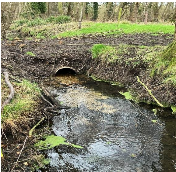
Before – Old culvert
