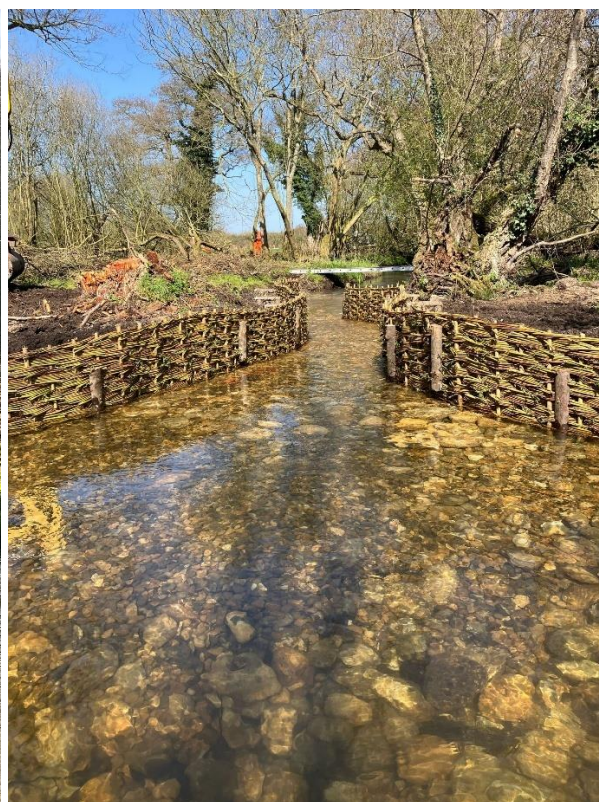
After - Fish/Eel Pass Installation
