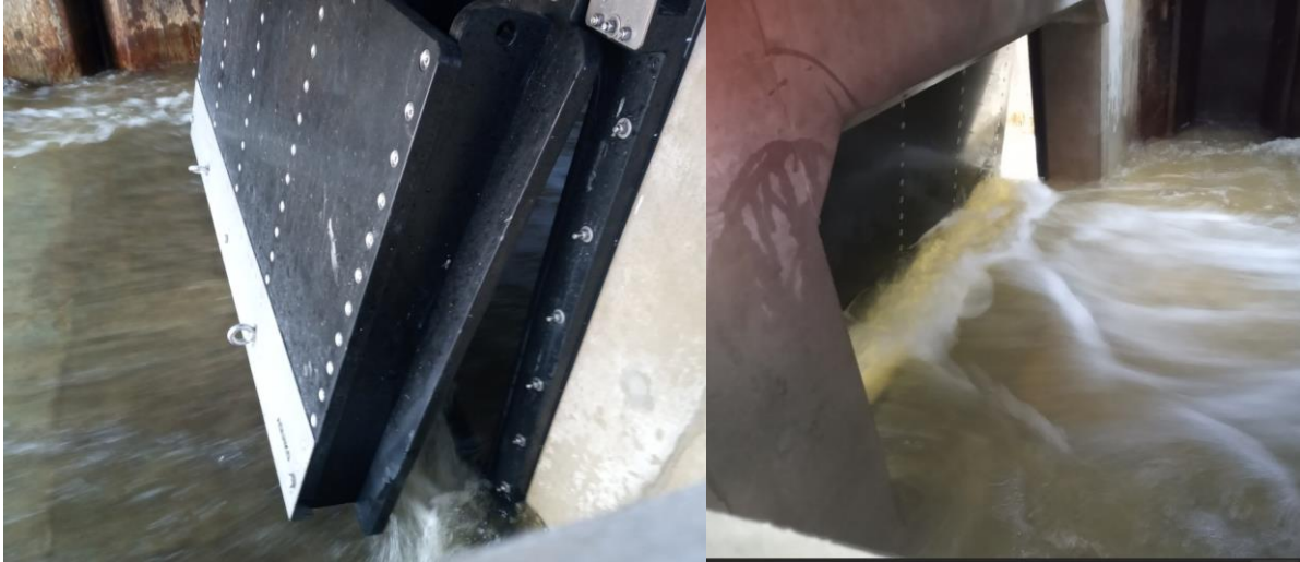
New larger flap valve not restricting water being discharged.
