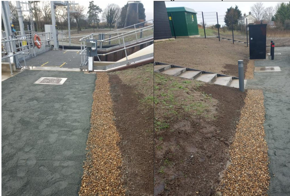
New French drain arrangement.
