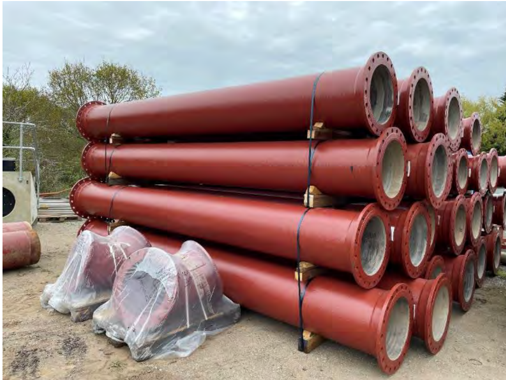
Ductile iron pipework at Martham for outfall replacements.
