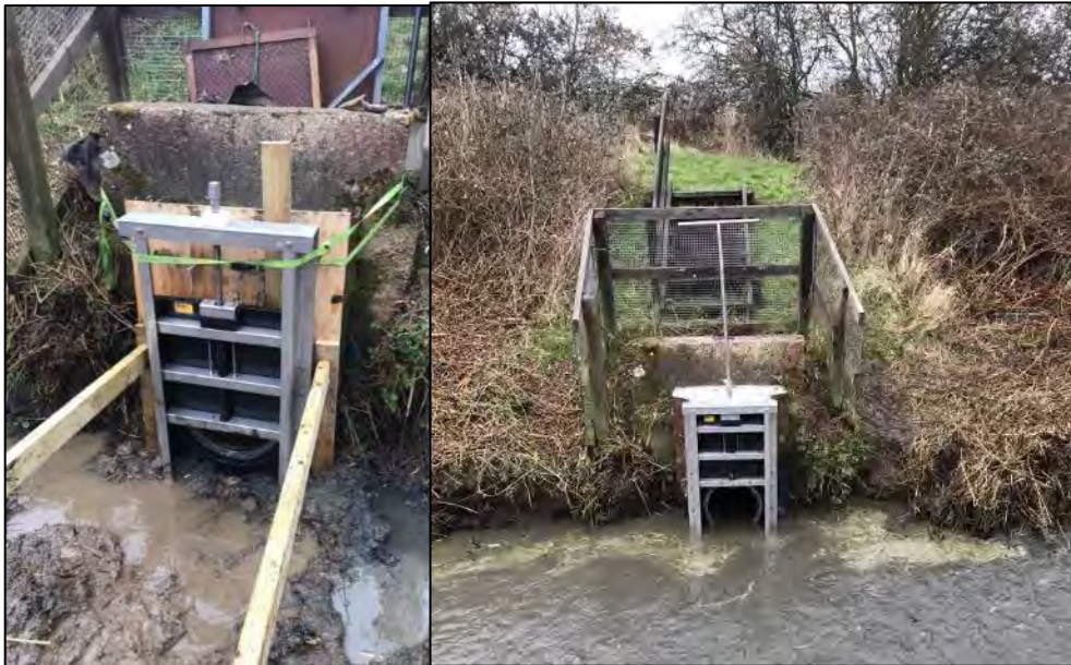
New penstock where board drains outfall into the EA main river
