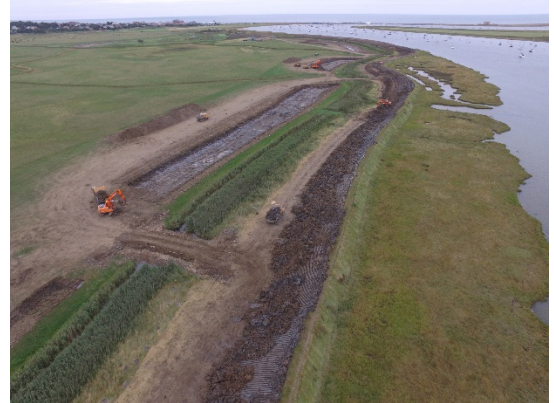
Aerial view of new soke dyke excavation early phases.
