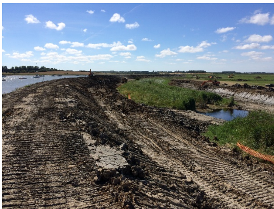
New widened bank at most downstream end of working area
