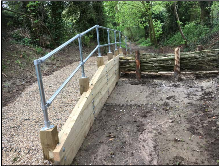
Close up of the new public bridleway structure beside the leaky dam.
