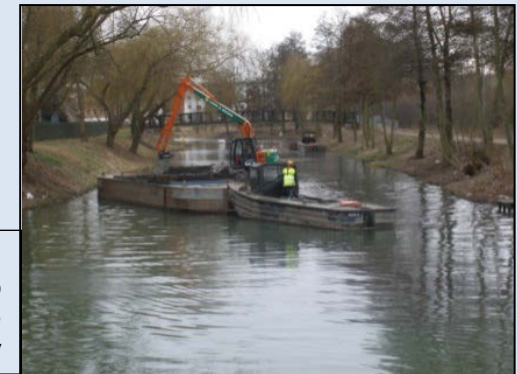
The barge-mounted excavator and skip barge ©Environment Agency
