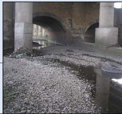
Gravel and silt accumulations at Chester Road Bridge, beneath junction 5 of M6 motorway ©Institution of Civil Engineers, 2014
