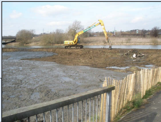
Land-based excavator removing material ©Environment Agency
