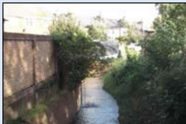
Concrete revetted channel of the Rags Brook ©Environment Agency
