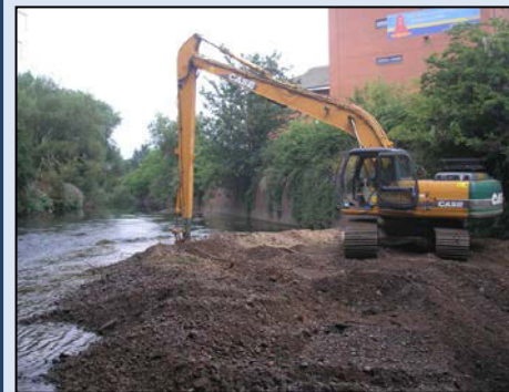
Gravel removal at Tameside Drive ©Institution of Civil Engineers, 2014
