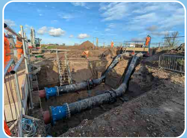
Above: Discharge pipework installed at St Benets undergoing leak tests
