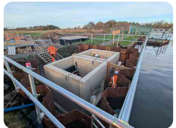
Energy dissipation outfall chambers installed at Horsey
