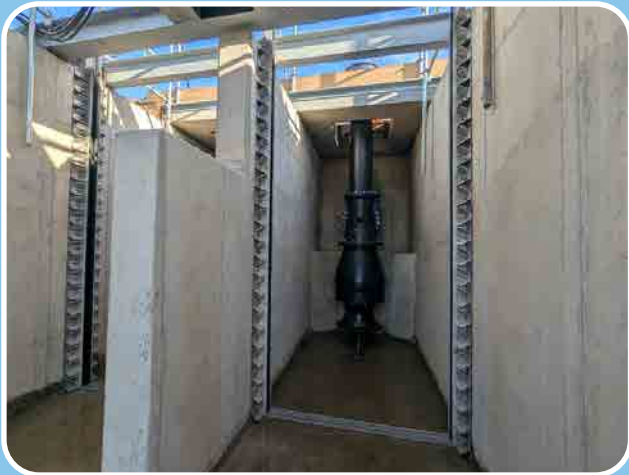
Above: St Benets wet well showing installed pumps, drop board slots, pump support slabs and steelwork
