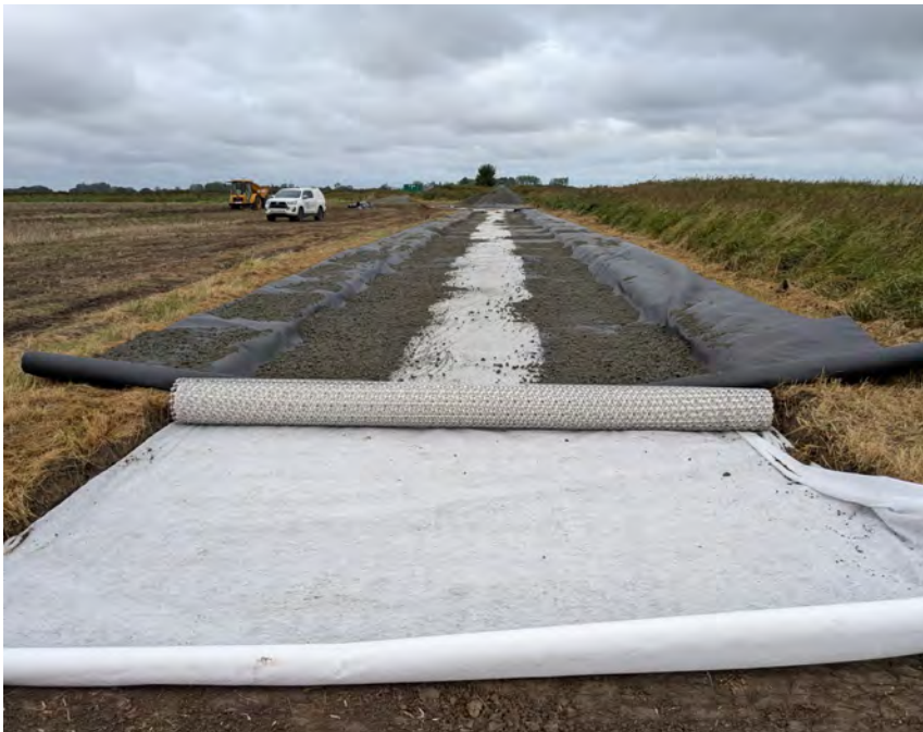
St Benets access track under construction
