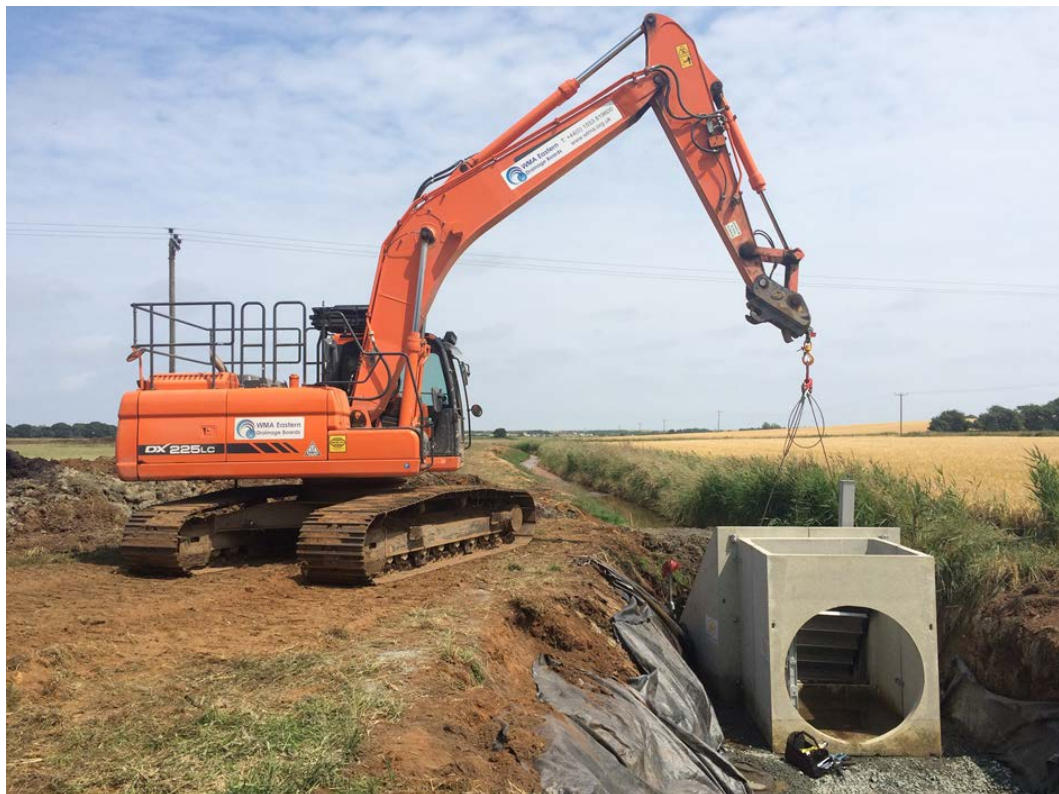
Composite stainless steel and HDPE plastic tilting gate being installed above
