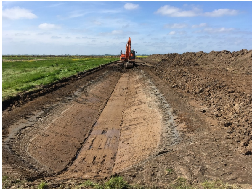
New soak drain being dug with specially made V bucket. Material being used to build parallel set back bank
