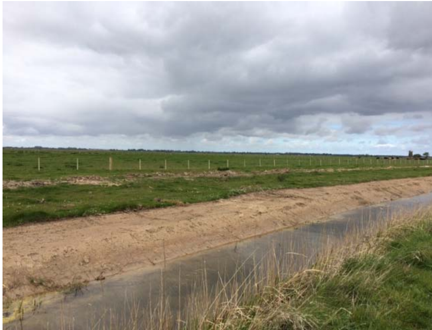
Water vole mitigation and fencing works at Halvergate
