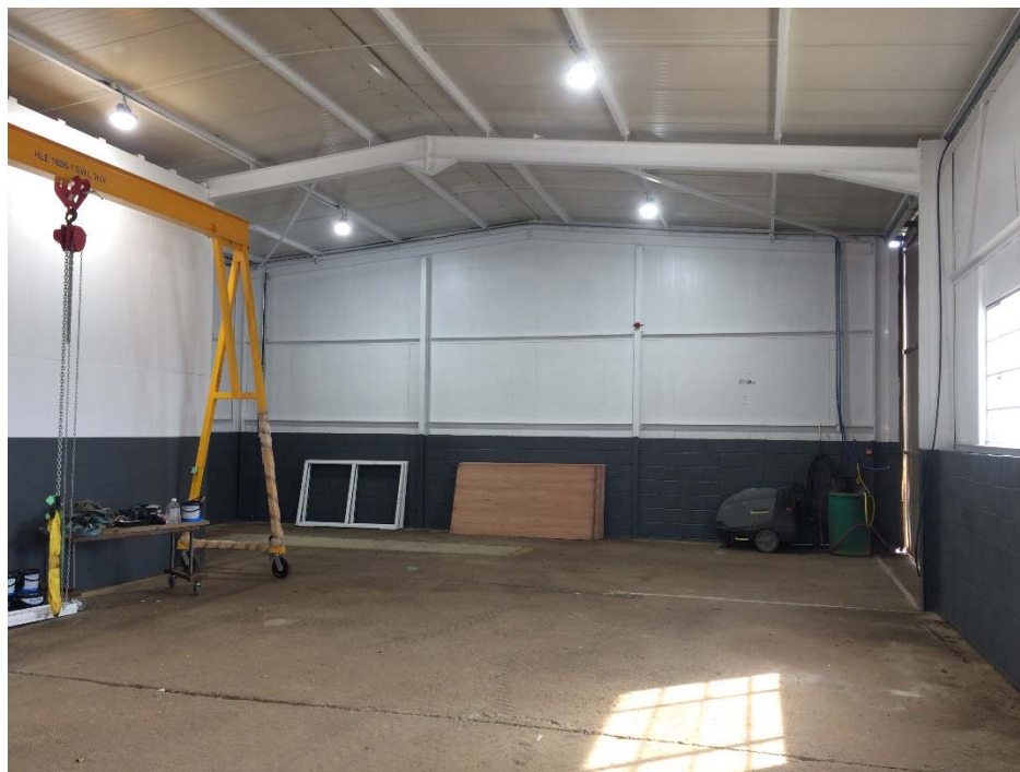
Workshop internal upgrades
