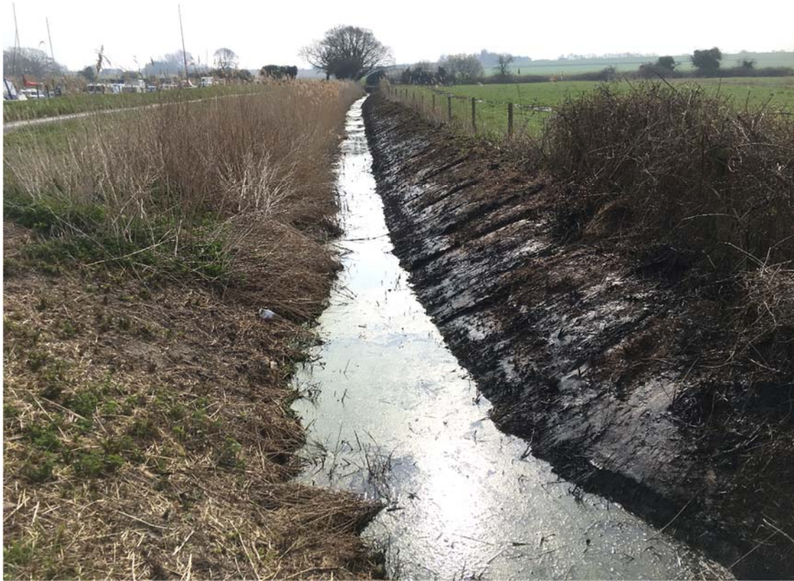
Water vole mitigation – bank has been flailed and scrape to displace water voles from one side of the dyke ahead of dyke widening.
