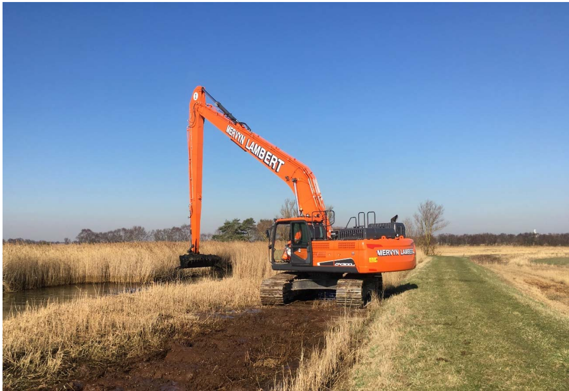
De-silting the Hundred Stream underway
