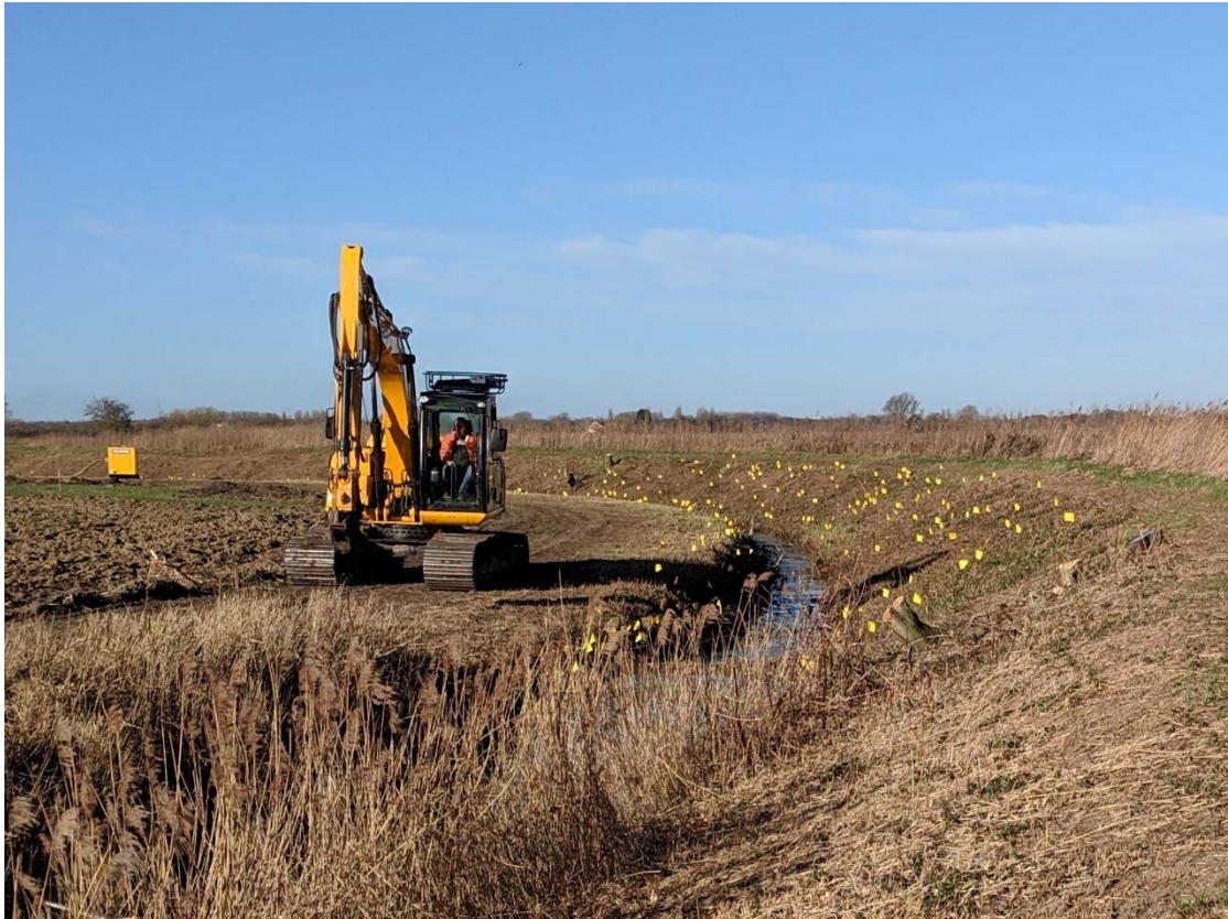
Water vole displacement mitigation on soke dyke with burrows marked by flags.
