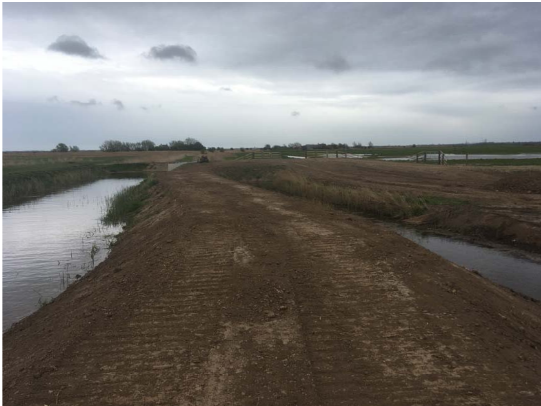
Newly constructed section of bank
