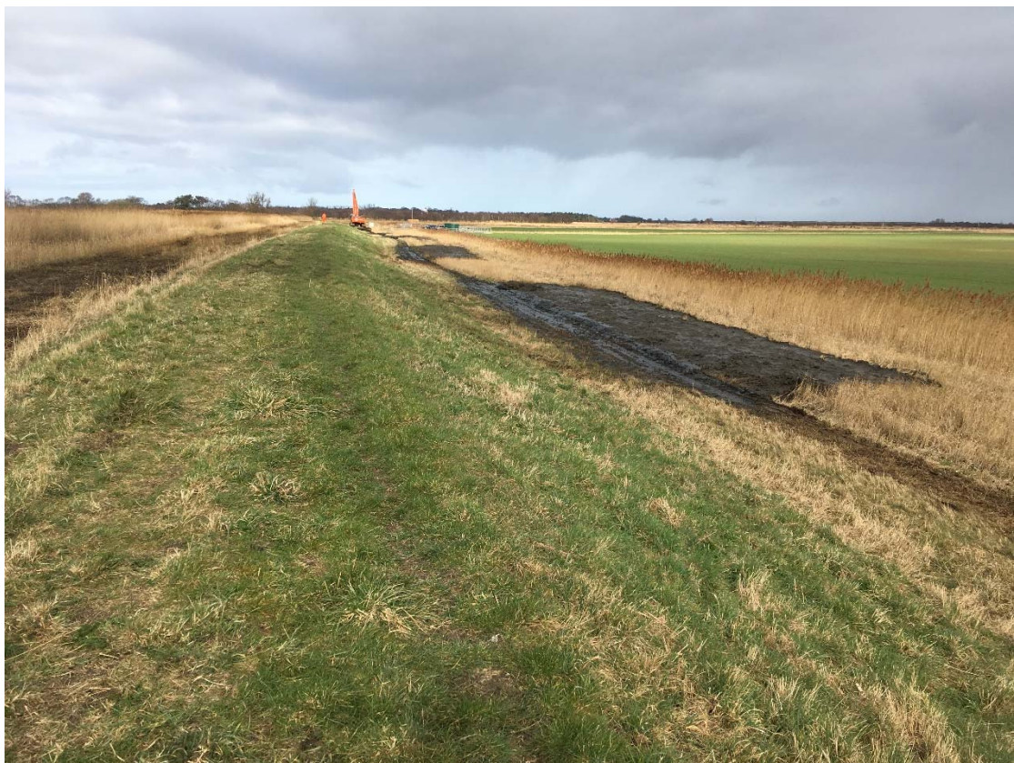
Silt removed from the bays in the Hundred Stream has been deposited behind the adjacent floodbank.
