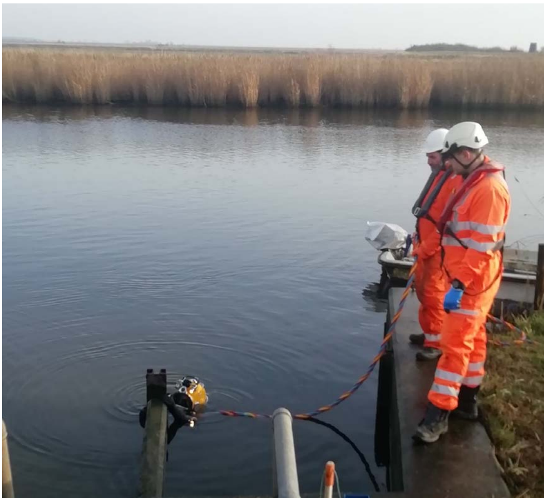
Photo showing diving operation to replace flap valves at Tunstall Pump Dec 19
