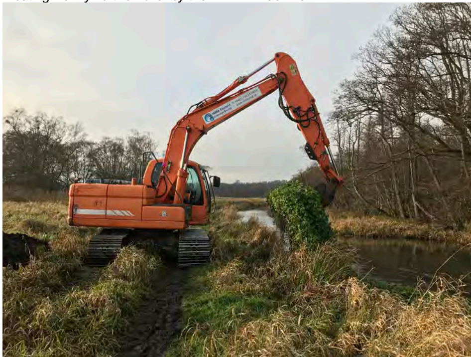
Floating Pennywort removal by the NRIDB Machine
