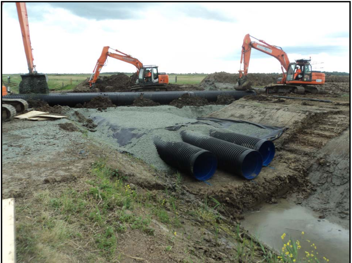
One of the new aqueducts under construction
