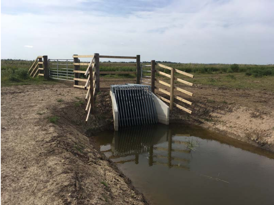
Completed auto-slucice structure
