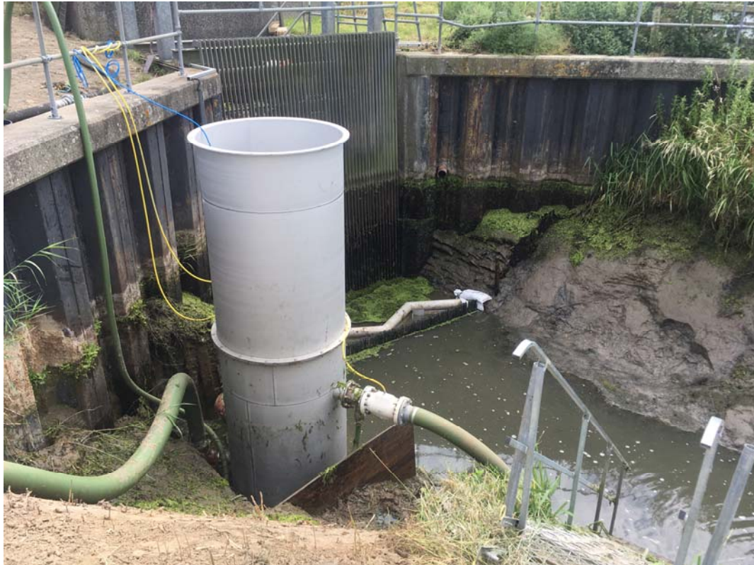
Installed tank, zig-zag inlet pipe and all other pipework
