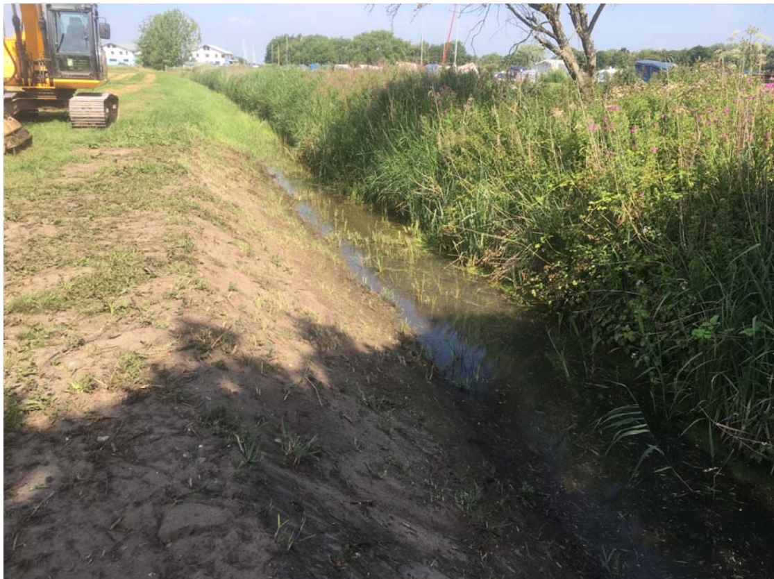
Water vole mitigation – continued flailing following displacement mitigation to maintain the habitat as unsuitable until works are completed.
