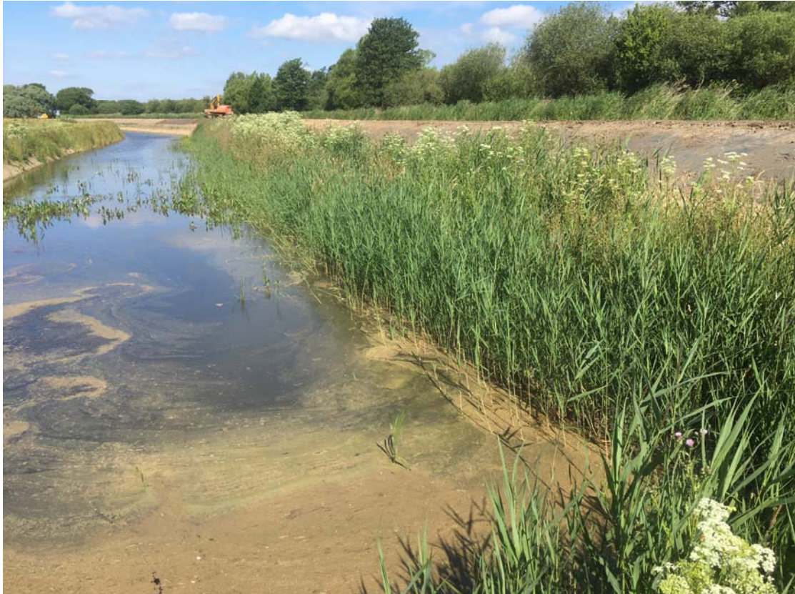
Vegetation establishing on new soke dyke completed in 2018.
