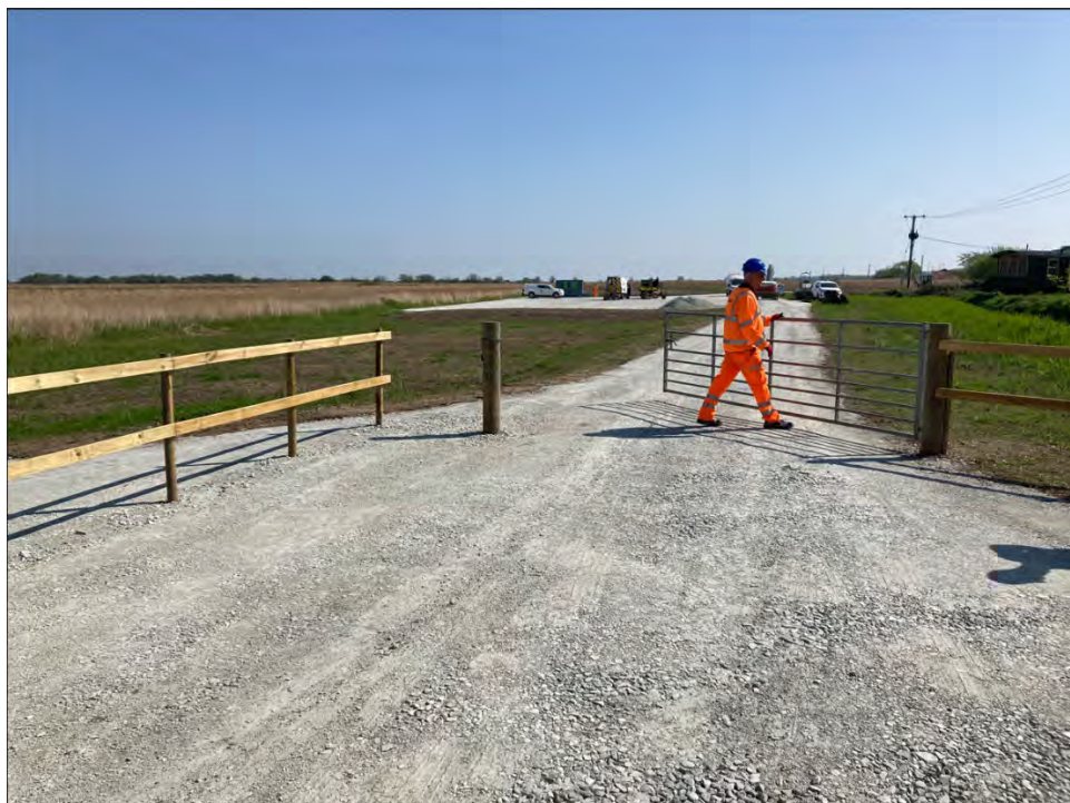
Reinstated fencing and gate at Potter Heigham, access track and contractors compound.
