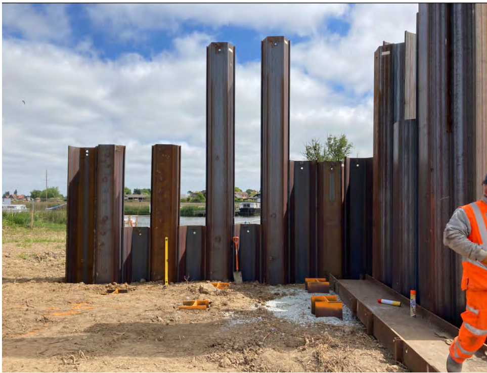
Installation of permanent H-piles and temporary sheet piles
