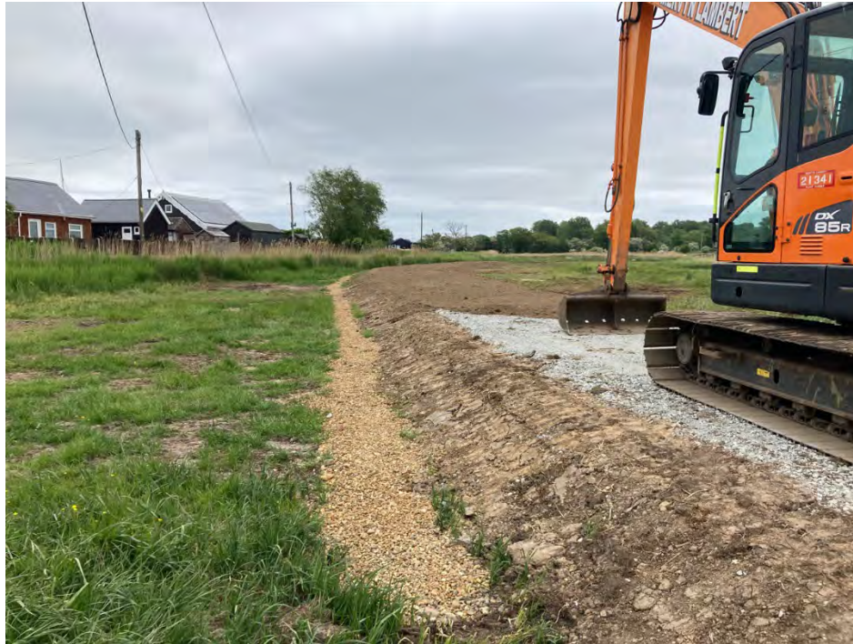
Permanent access track in construction, French drain installed to prevent pooling
