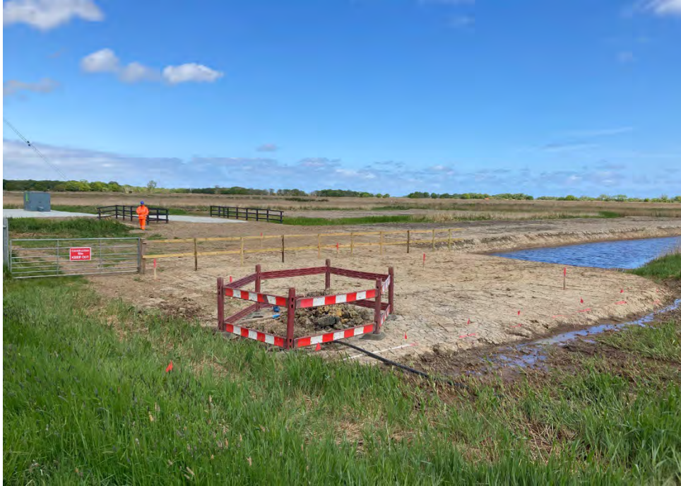
Completed culvert, reinstated fencing, drain works and UKPN cabling.
