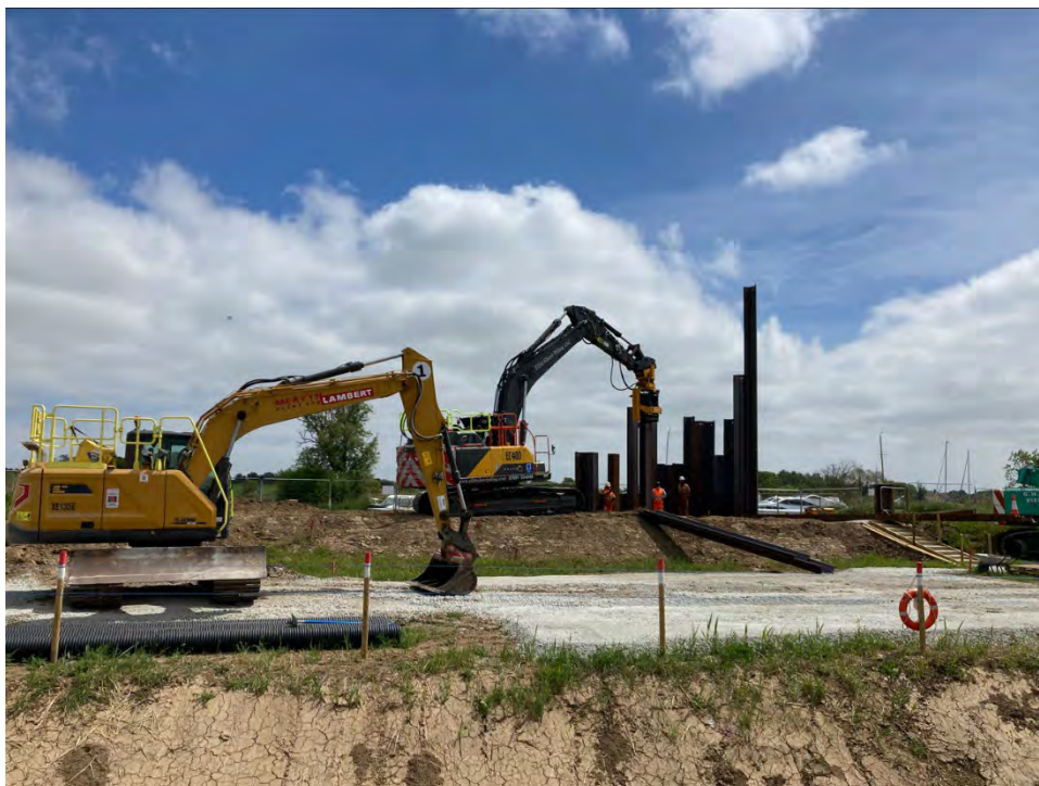
Installation of H-piles and temporary sheet piles
