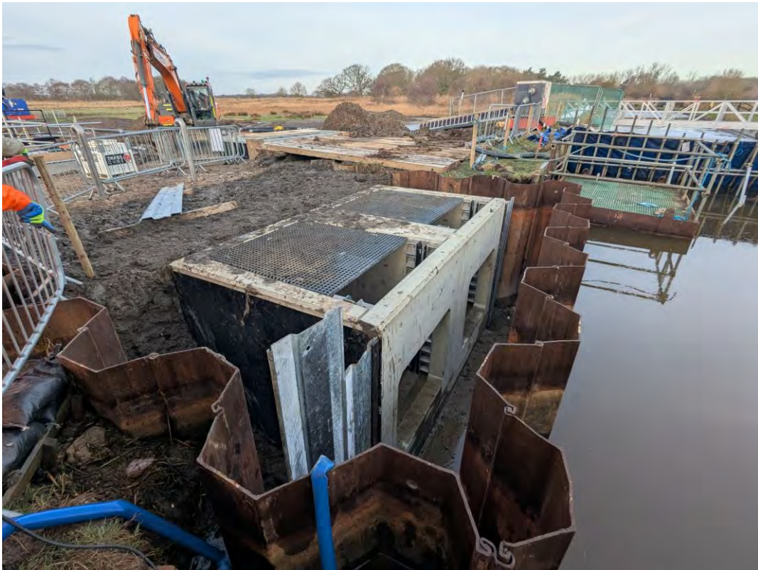
Horsey outfall structure prior to temporary pile removal
