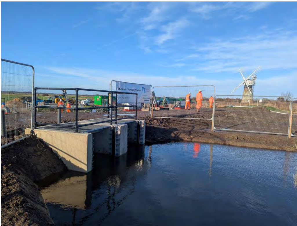
St Benets outfall structures and reinstated flood bank
