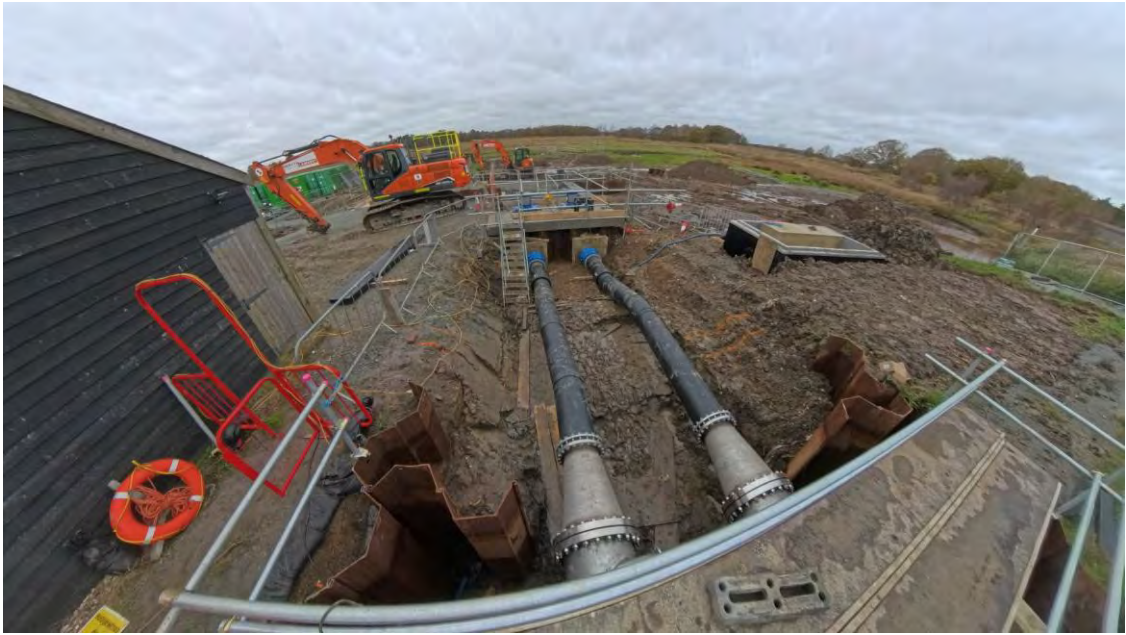
Horsey discharge pipework during installation
