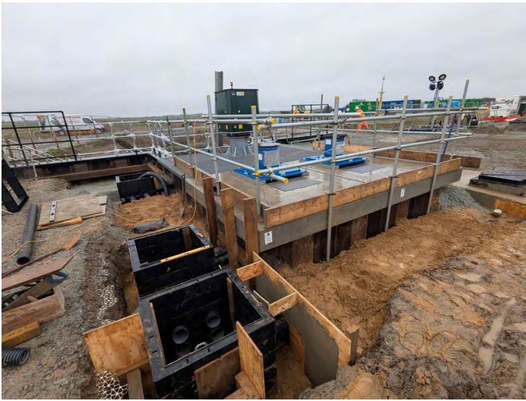
St Benets draw pits / cable ducting installation
