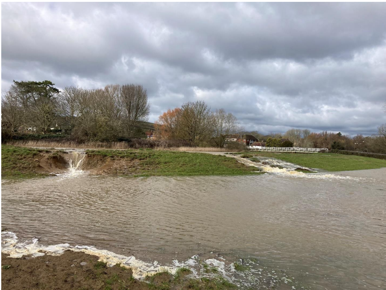
Figure 6-3: Overtopping of the River Cuckmere at eroded sections of embankment (credit: PCWLMB).
