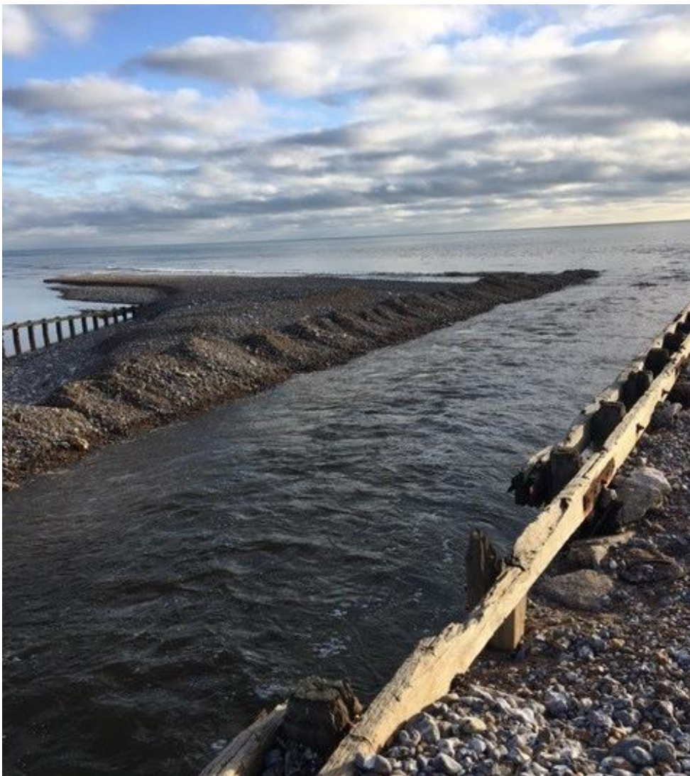
Figure 3-3: Timber training walls through shingle beach at mouth of River Cuckmere (credit: PCWLMB)
