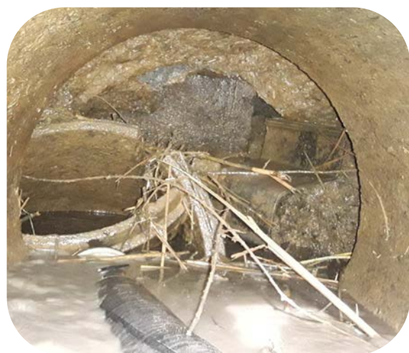
Barsham Culvert in poor condition
