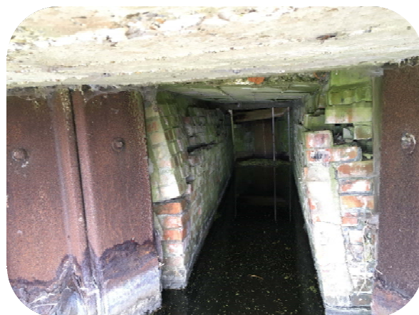
Short Dam wet well in poor condition
