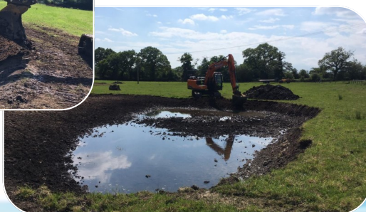
Right: Newly deposited berms, encouraging gravel scour
