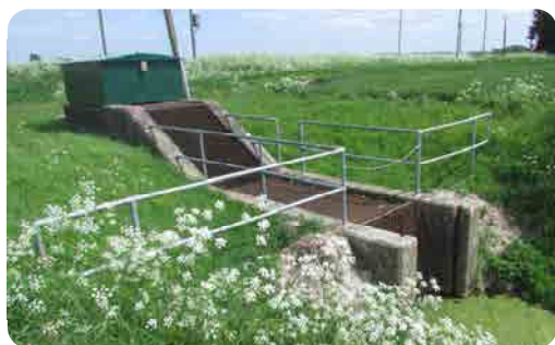
An Archimedes screw pump
