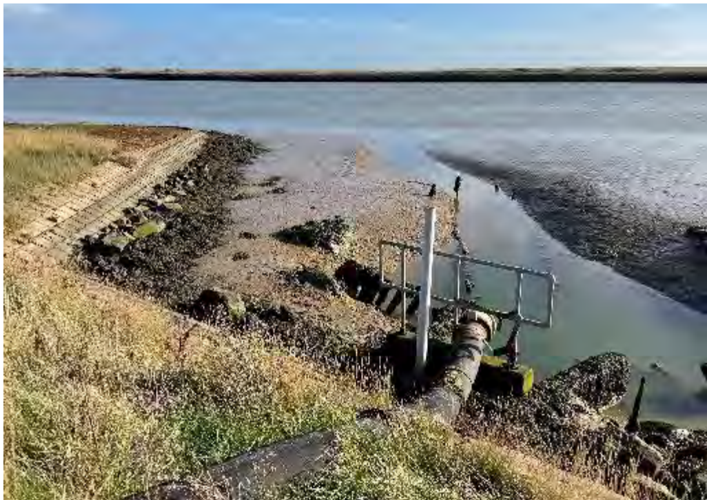
Gedgrave Pumping Station outfall. Current temporary pipework over the flood defence.
