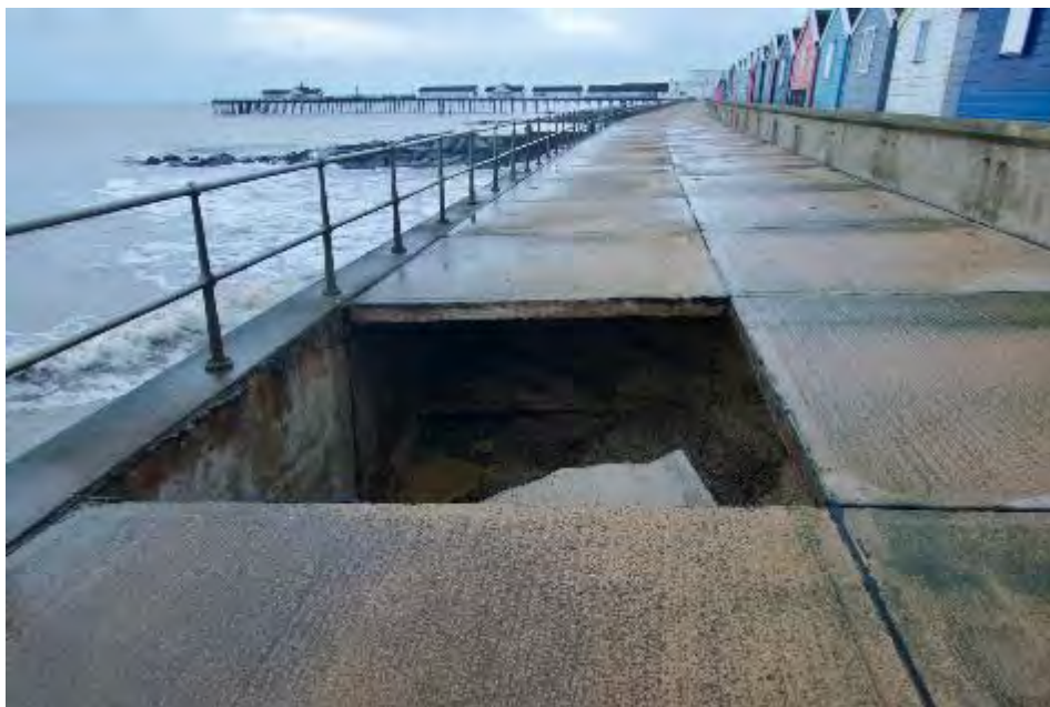
Voiding and slab collapse on Southwold promenade
