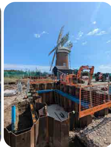
Factory testing of one of the new Horsey pumps & Horsey pumping station wet well in construction
