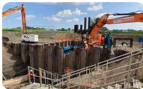
St Benets pumping station wet well - temporary piling can be seen in the background
